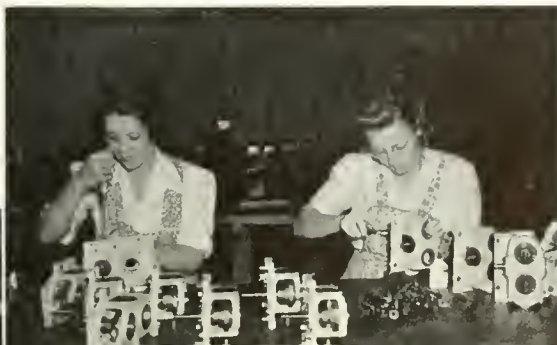
LEFT: ONE OF THE THOUSANDS OF GOVERNMENT-ORDERED 16 MM. PROJECTORS IS SHOWN ON THE INDIANAPOLIS ASSEMBLY LINE; BELOW: SOUNDHEAD GEAR BOX SUB-ASSEMBLY AND HIGH-POWER AMPLIFIER EQUIPMENT RECEIVING FINAL TOUCHES BY GIRL EMPLOYEES.
